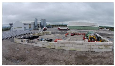
Cenin Renewables uses nearly 3000 PV panels producing over 735kw as the main power source for parent company, Cenin Cement, and to feed into a 400 kw grid connection. With sustainability at the heart of their cement manufacture, they are in the process of installing an on-site wind turbine and have plans for anaerobic digestion and a 1MW PV solar trekker system.
