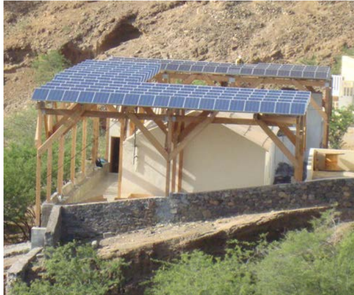
Figure 24. Pergola installed in Cabo Verde by TTA (source: TTA)
